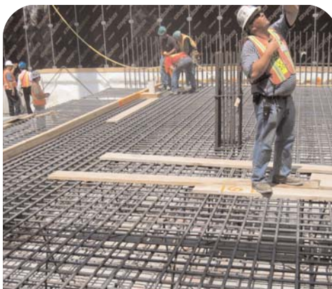
Matty Smith directing the rebar installation at the invert station area.
