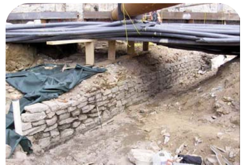
Third historical wall, about 105 feet long and nine feet thick, believed to have been a sea wall. This wall, unlike the previous two recently discovered, has barnacles and oyster shells stuck to it.
