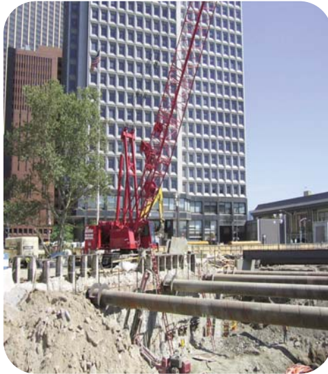
Manitowac 777 Lattice Boom Crane at south excavation
